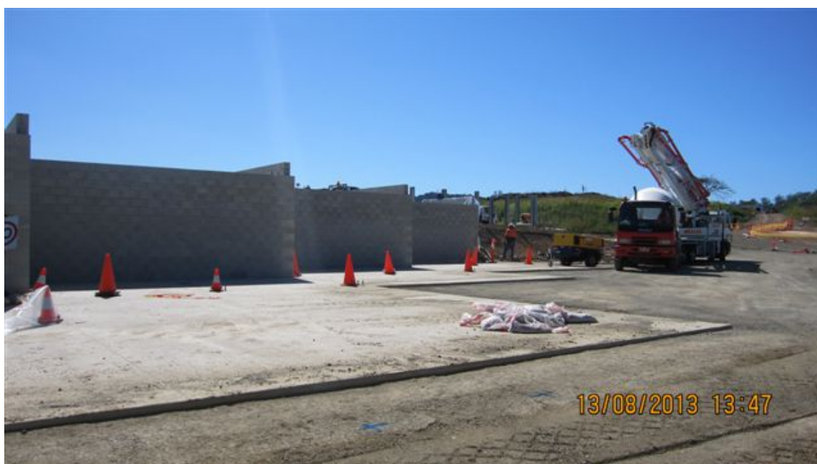
Figure 3.3 Construction of new transfer station at the former Sarina landfill (August 2013)
