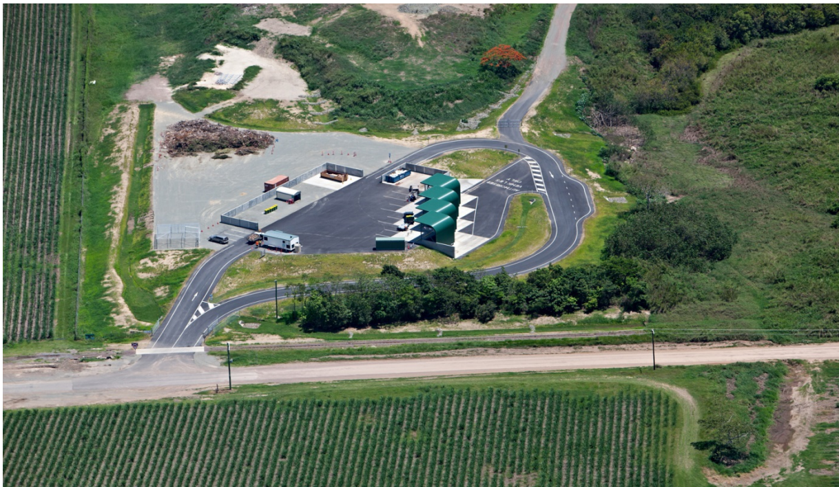
Figure 3.2 New transfer station at the former Sarina landfill
