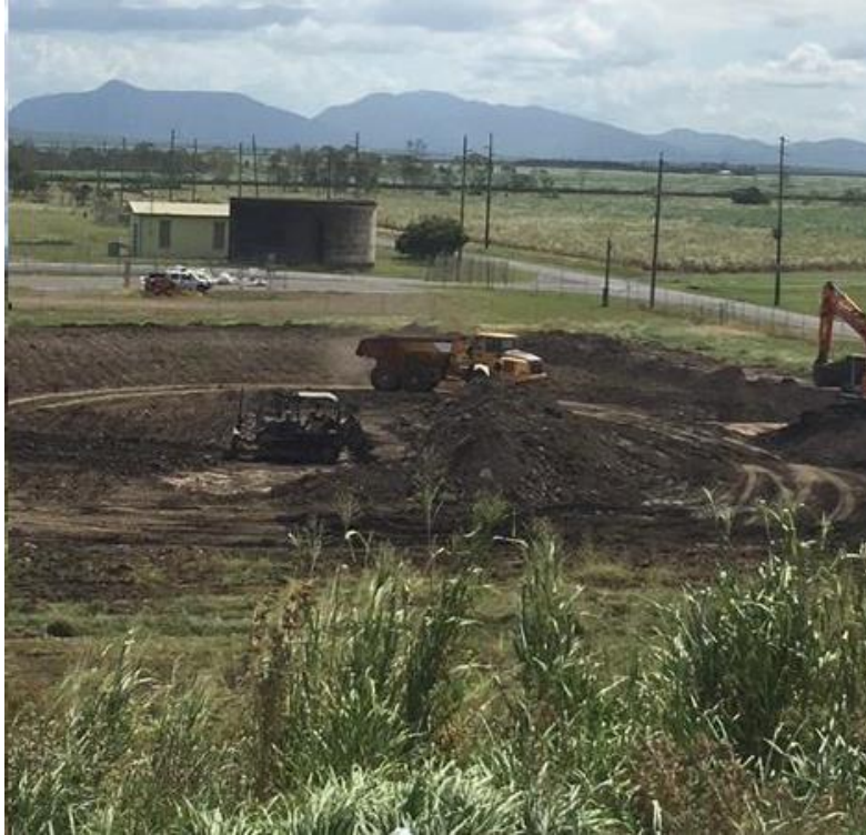
Kelsey Creek Landfill cell 5 construction
