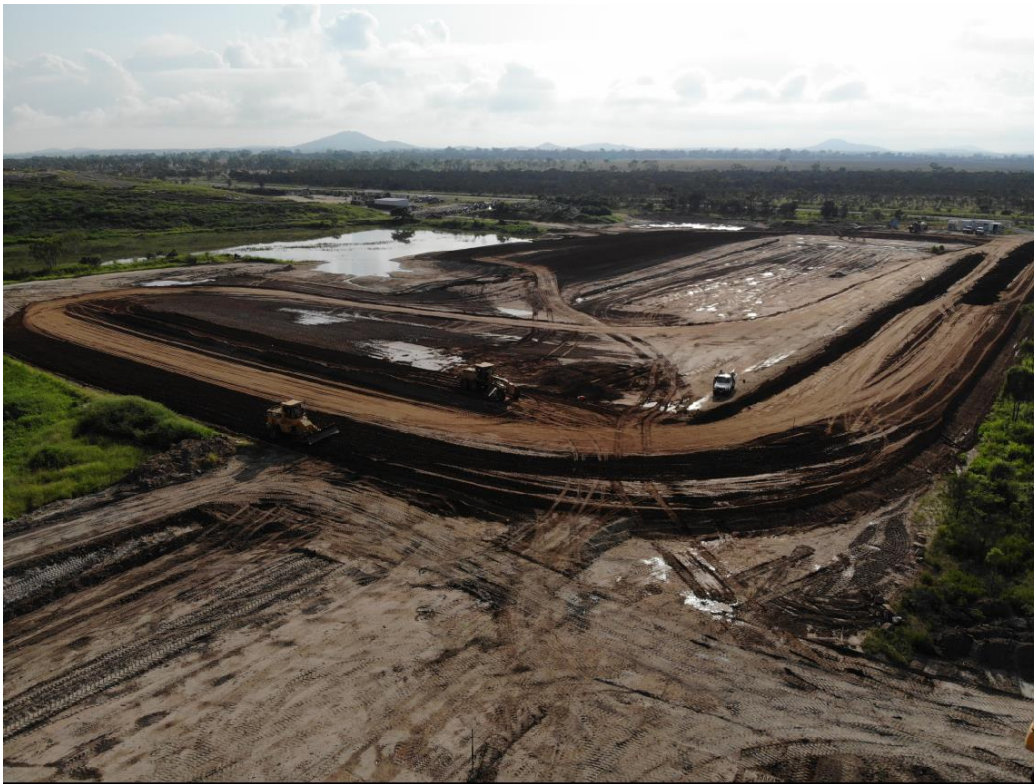
Bowen Landfill cell 6 construction
